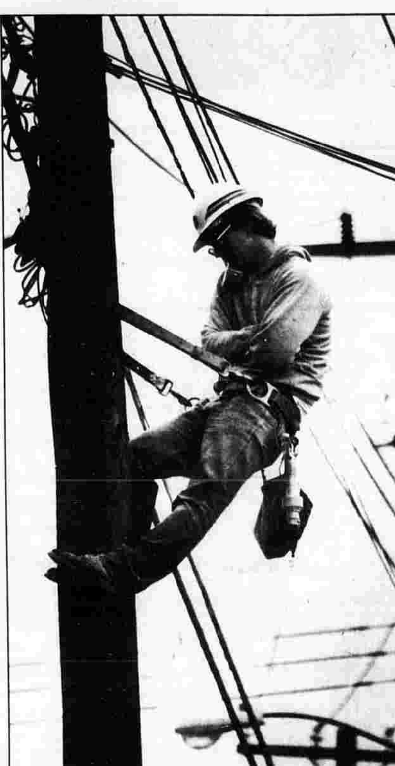
LONG DISTANCE — Bill Hahn, a service technician with SNET, makes a phone call the hard way Thursday while working on Spruce Street. He was calling a customer to tell her that a new line had been connected and her phone was working.
